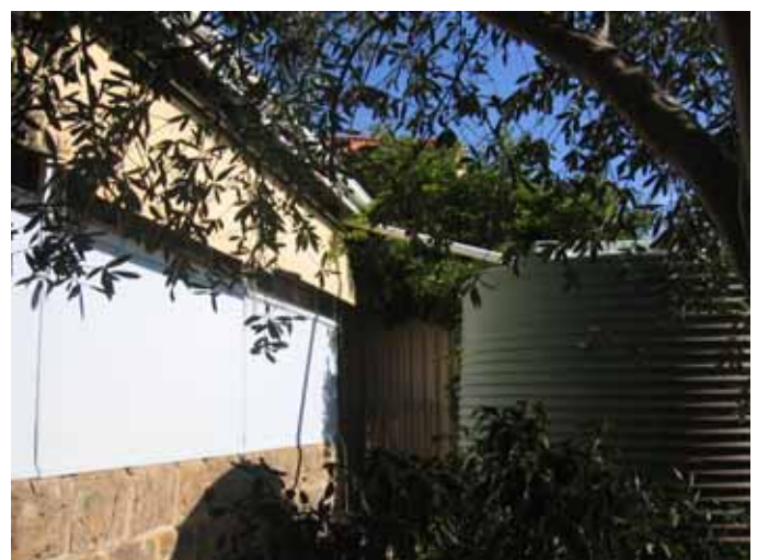
West frontage; (hottest side) blinds, vegetation, water tank yet to be plumbed into house.
